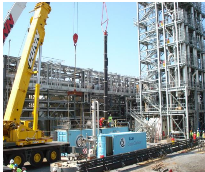
MTU being installed next to PSTU
